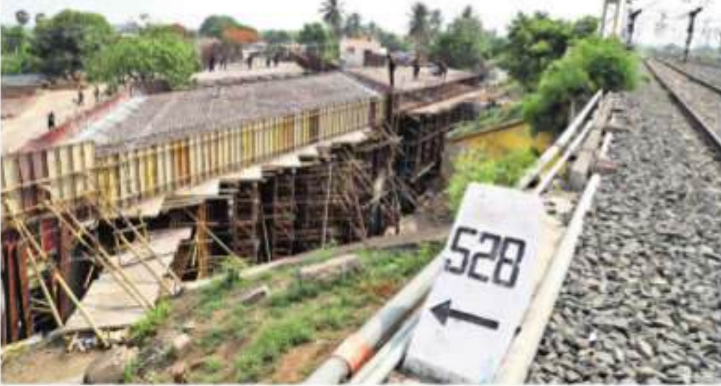
Work under way for the new railway underpass in Coimbatore | S SENBAGAPANDIYAN
